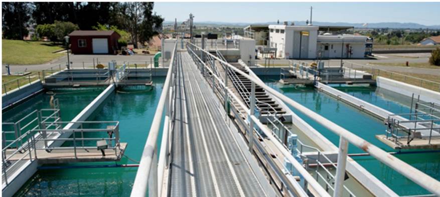
Travis AFB Water Treatment Plant
