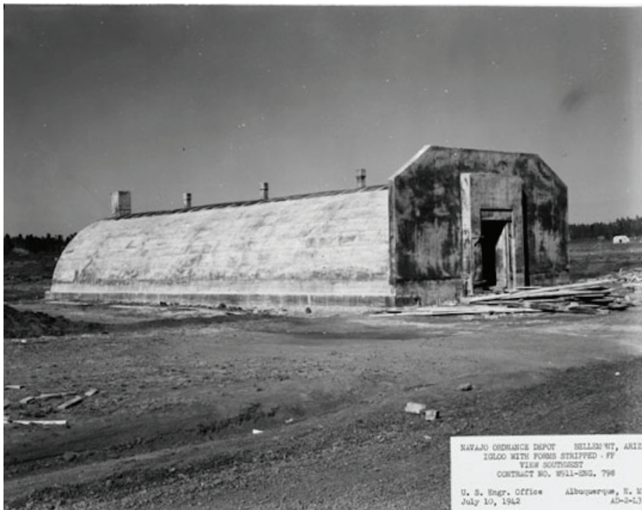
FIGURE 2.05 Ordnance igloo being constructed in 1942 (Source: Camp Navajo, Army National Guard, 2018)
