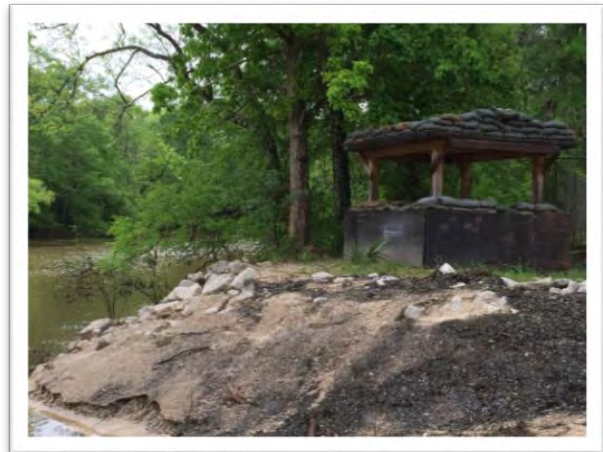
Figure 28 Facilities used for training within the WMA
