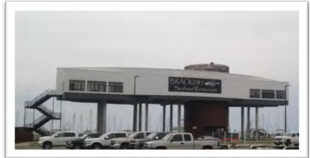
Figure 15 New construction in Gulfport (above) and Long Beach (below) depicting the additional construction standards after Hurricane Katrina
