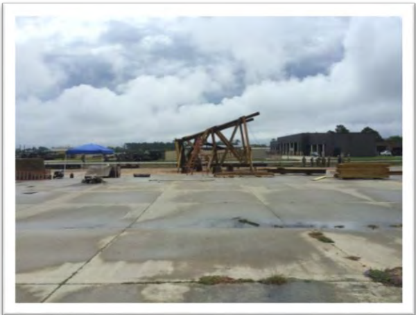
Figure 25 Construction training exercises
