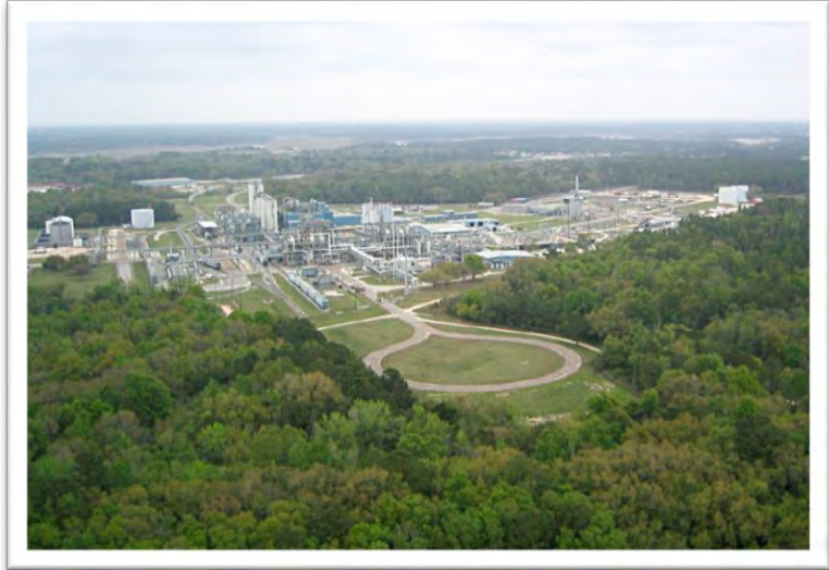
Figure 20 Overview of Port Bienville
