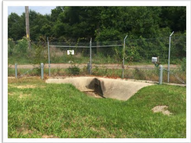
Figure 53 Drainage canal located within NCBC Gulfport
