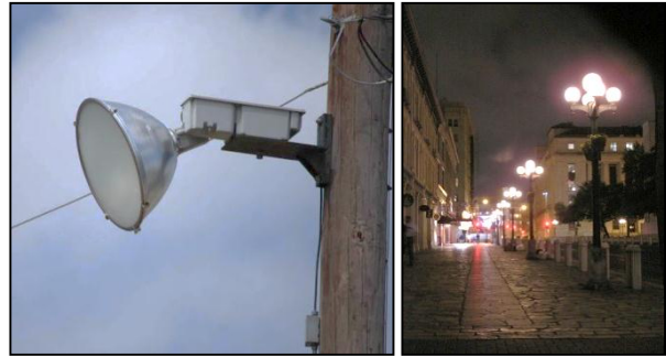
Examples of poor street light fixtures that result in light spreading past where it is needed, and creating excess ambient light
